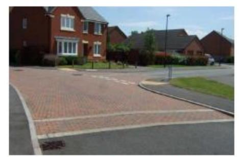
Raised Table in Block Paving with Tactile Paving at Crossing Point
