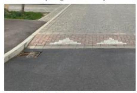
Raised Table in Block Paving Detail
